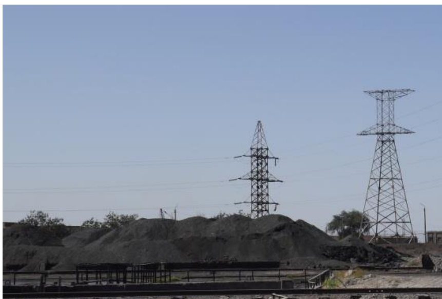
Figure 9.4.7 Site for temporary disposal of dust from the gas treatment system's bag filters at ESMS
